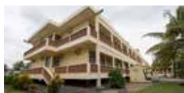
Hospital Out-Patient Extension (HOPE) Center Hospital Ward Refurbishment, Antananarivo, Madagascar
